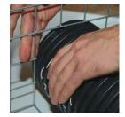
Push through the Runaround Pipe two ridges in. Tease it in for a snug fit.
